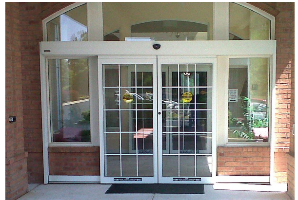
SURFACE APPLIED AUTOMATIC SLIDING DOOR
